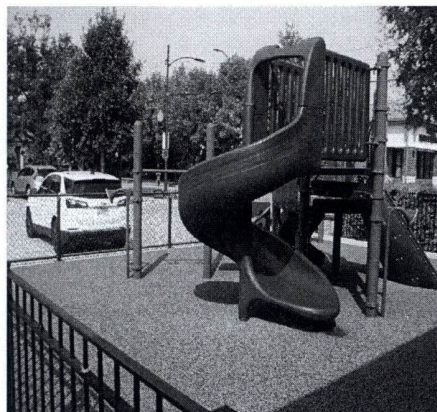
Existing playground with PIP rubber surfacing
